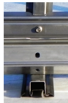
One common bolt for all joints
