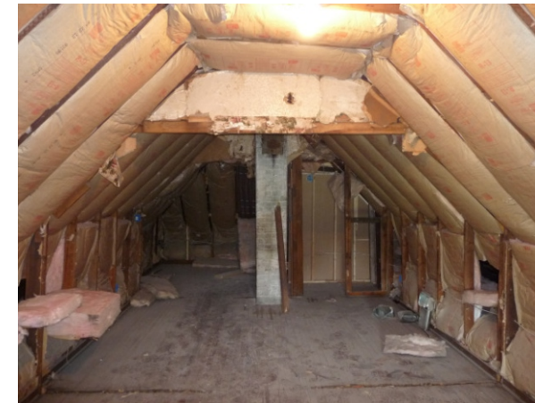
KNEE WALL SUPPORTS IN ATTIC
