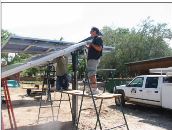
Lifting and bolting the sub-array onto the tube.
