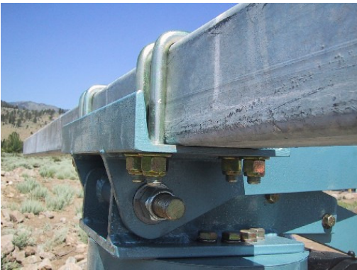
TIGHTEN NYLOCK 5/16" U-BOLT NUTS EVENLY .
