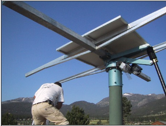
Module Rail & Support Angle Detail From the bottom
