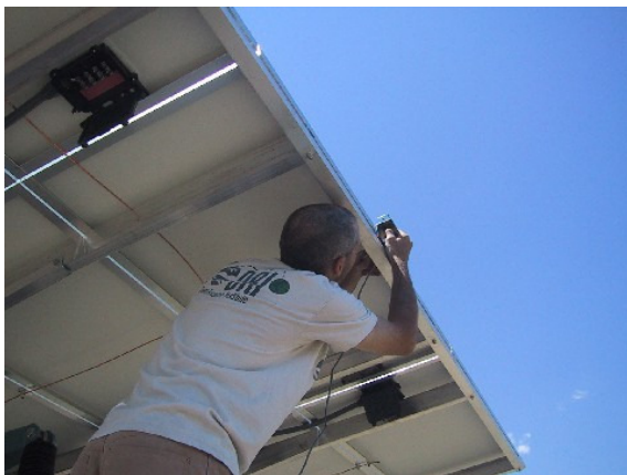
Sensor mounts on the top edge of the array. Center it on the top makes for a neat wire run. The remote sensor wire plugs into the base of the sensor. Twist the lock ring!
