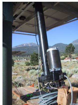
If you have the Dual-Axis Option: There is a two-wire "pig-tail" that is prewired into the azimuth motor. It needs to be connected to the elevation actuator motor.
