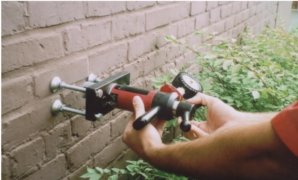
Hilti pull test on east anchor
