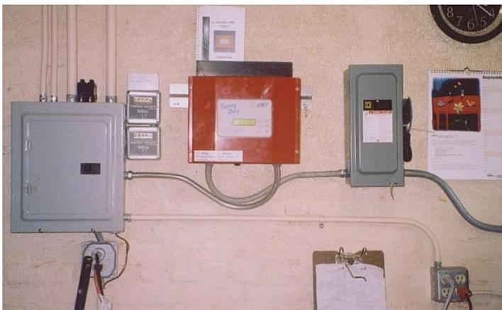
project was finding out that direct current (DC) arcs more easily than alternating current (AC). Therefore the Disconnect had to be a special DC disconnect, and the positive wire had to be split across two blades of the switch to prevent arcing.
