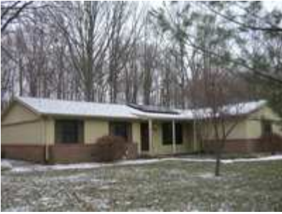
1.9 kW Electric System Plymouth, MI
